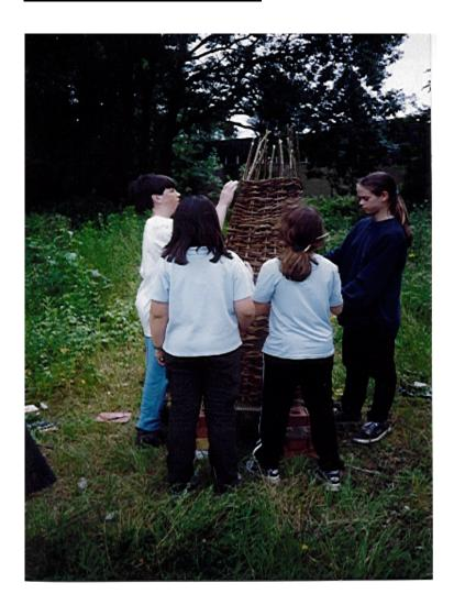
The clay kiln is constructed on a willow and hazel structure. The structure has the shape of a tapering chimney, measurements at base of chimney is 3 ft Diameter made with 8
